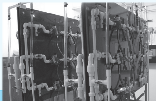
At left: Pipe loop testing simulates conditions found in service pipes and home plumbing.
