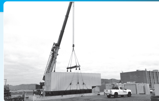
The third generator before and after being set into place
