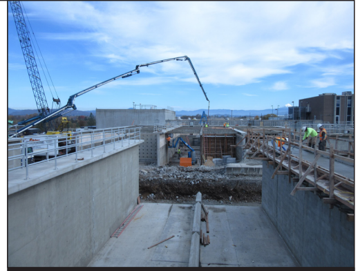
Expansion project ongoing
