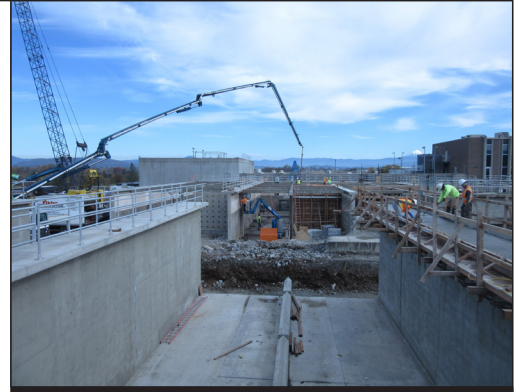
Expansion project ongoing
