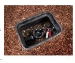
Between irrigation cycles, look for areas of the landscape with water pooling on the surface, which could indicate an underground leak. Check the valve boxes that house controls and other components underground to make sure that valves are securely connected and can close completely, so they do not slowly seep water even when they are turned off. Installing a flow meter can also help you know when your system has a leak.
