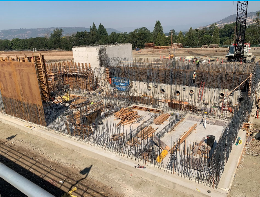
Duff Water Treatment Plant Filters Construction
